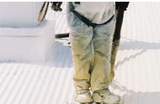
BASF protective coating
