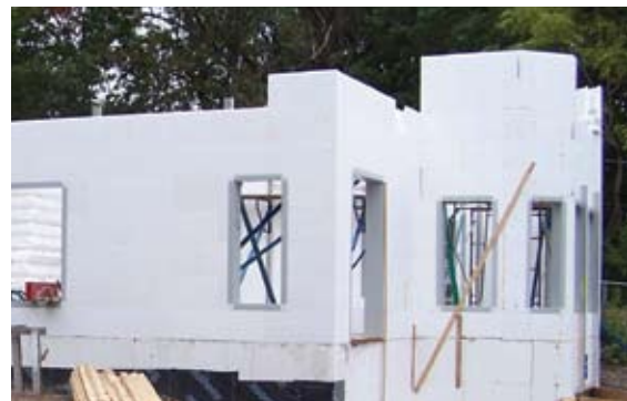
Insulating Concrete Forms (ICFs)
