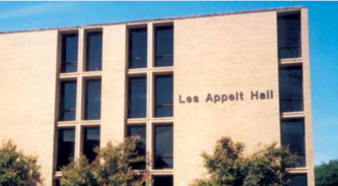
The main Texas A&M University campus boasts over 7 million square-feet of SPF roofing.
